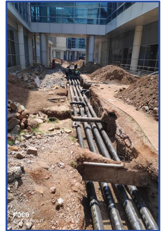
Holiday test of Anticorrosive wrapping coating and Pipes laying
